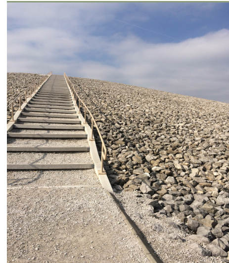
02 Steps to Weldon Spring disposal site. Photo: Thomas Turnbull.
